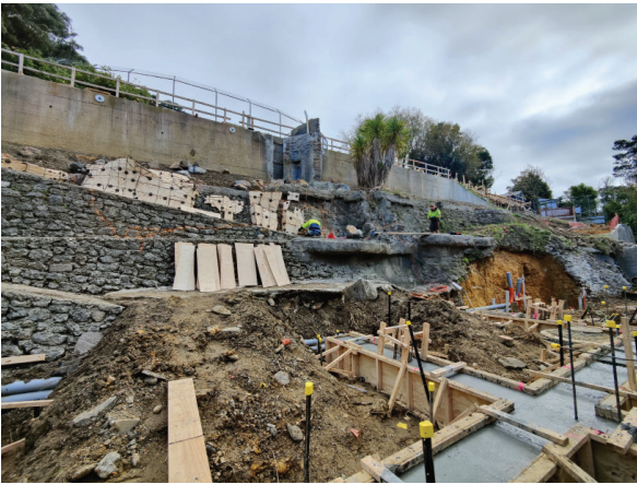
Construction progress so far
