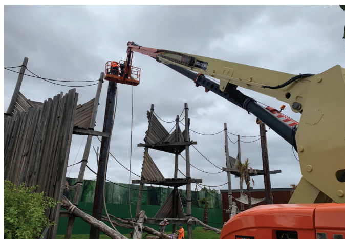
Construction work at Sydney Zoo
