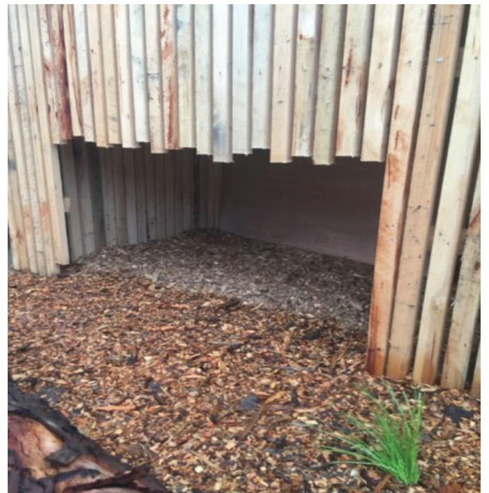
Figure 2: One of the lock-aways
