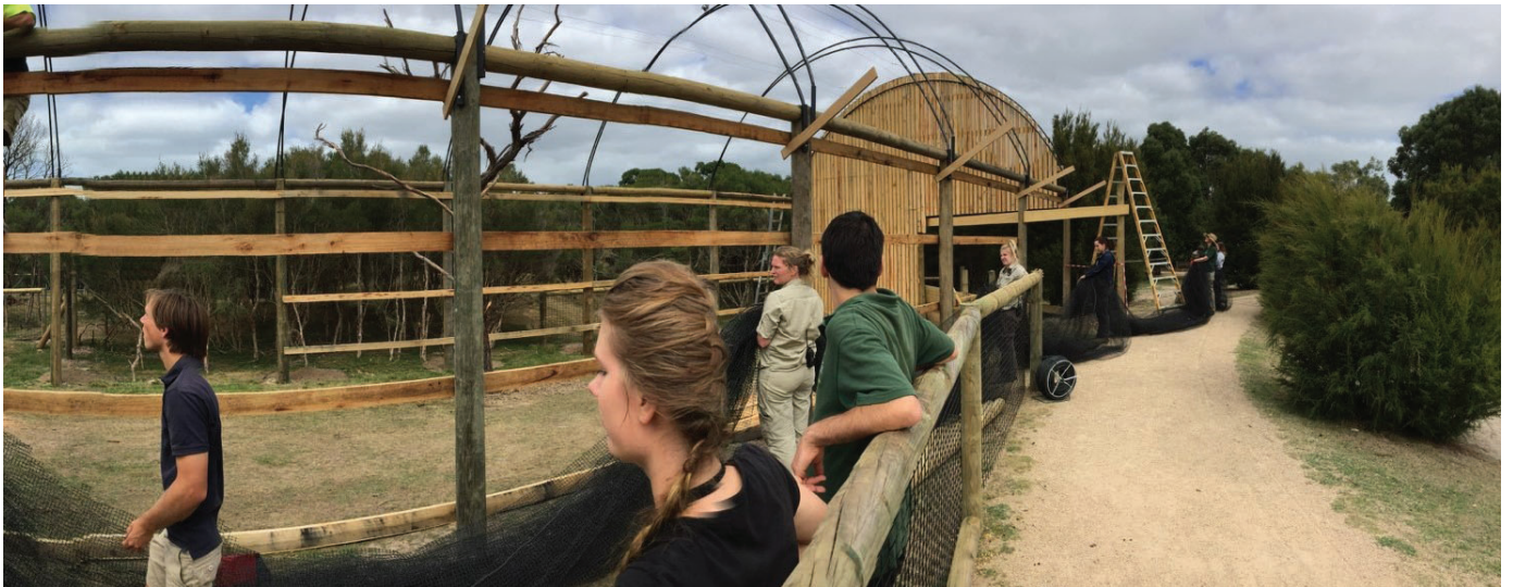
Figure 1: Building process of the Wedge-tailed Eagle aviary
