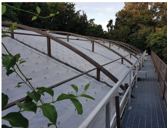
Butterfly House roof with double paned glass, showing the open and close positions of the shade cloths
