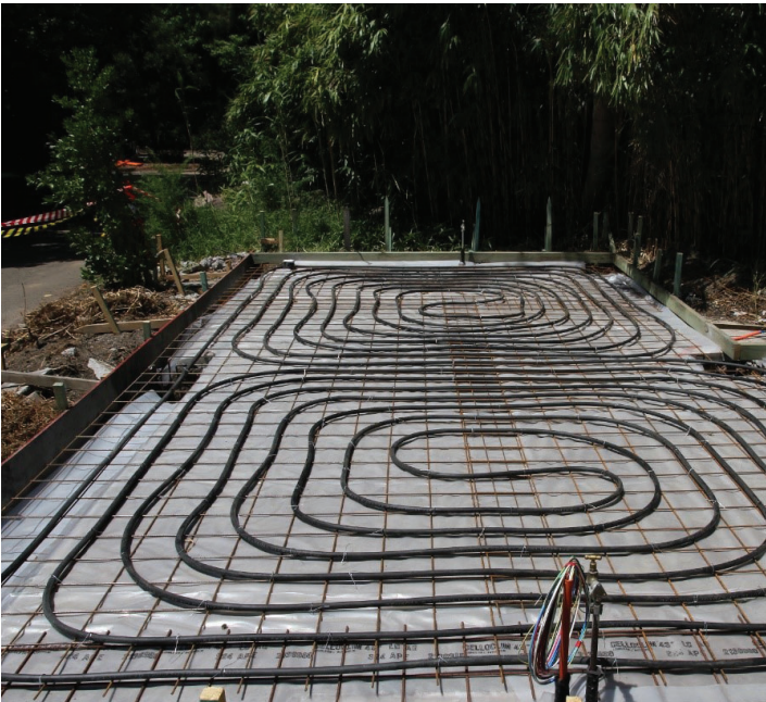
Underfloor hydronic heating coils before concrete was poured over the slab
