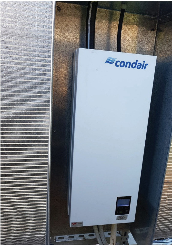
Inbuilt hot steam humidifiers, Condair CP3 Mini
