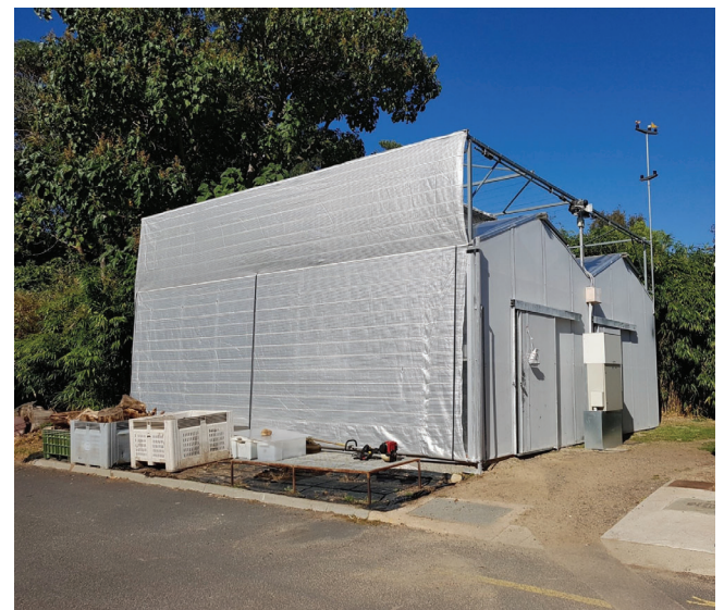
The LHISI glasshouses reflective shade cloth (Svensson 80% Shade)
